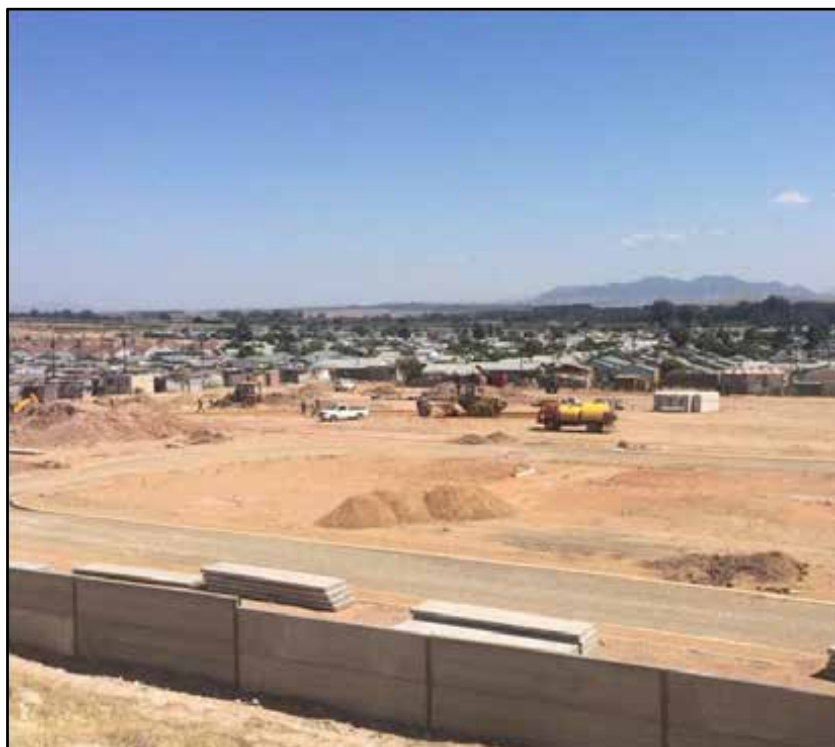
Installation of services in progress.
